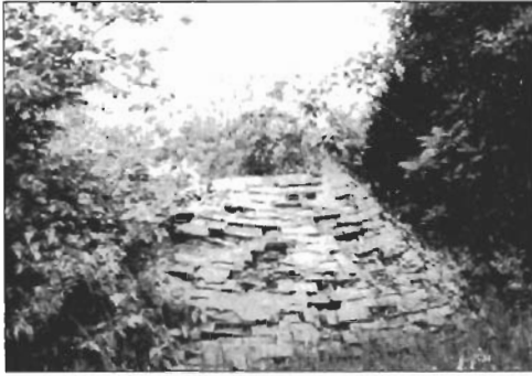
Figure 1. — Above-ground portion of cistern used for nesting by Eastern Phoebe.
